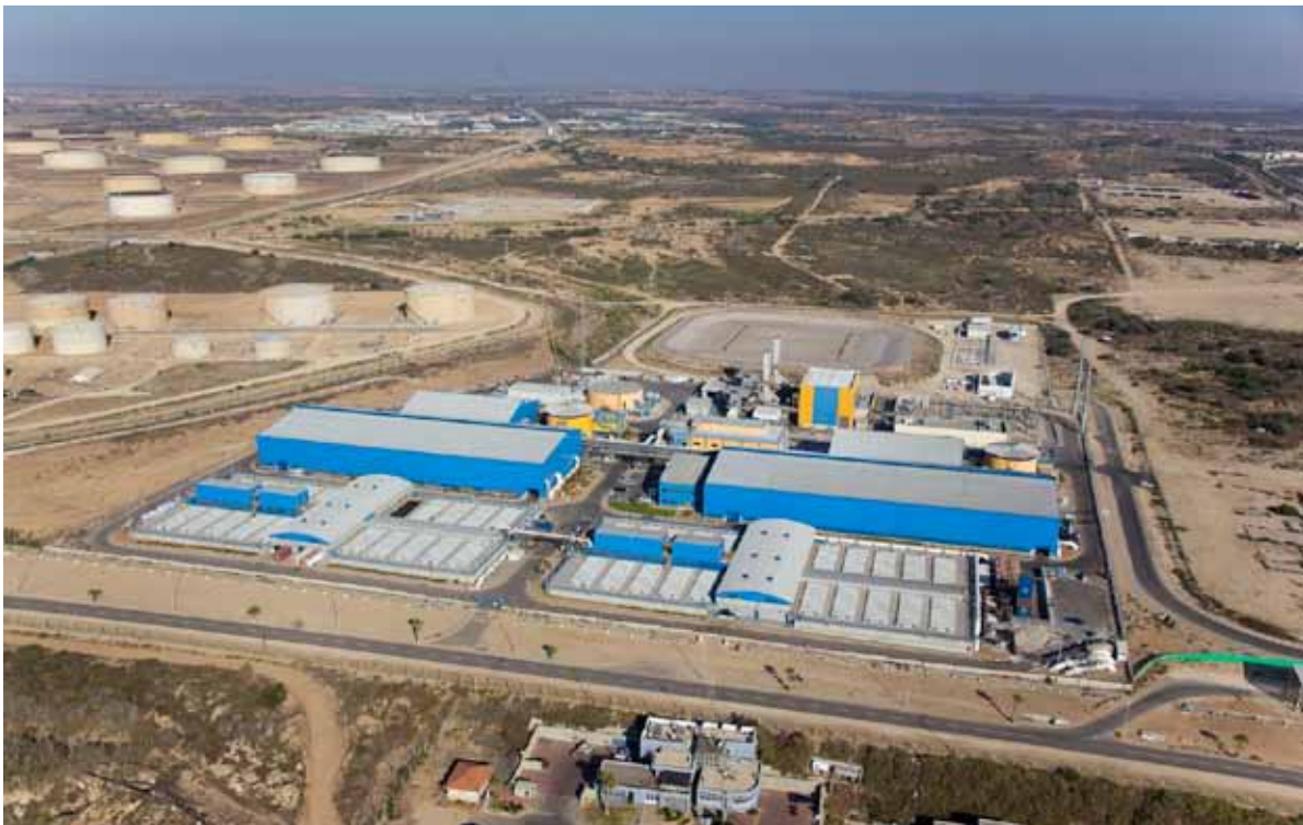
Fig.6.5: Desalination Plant at Nemili
